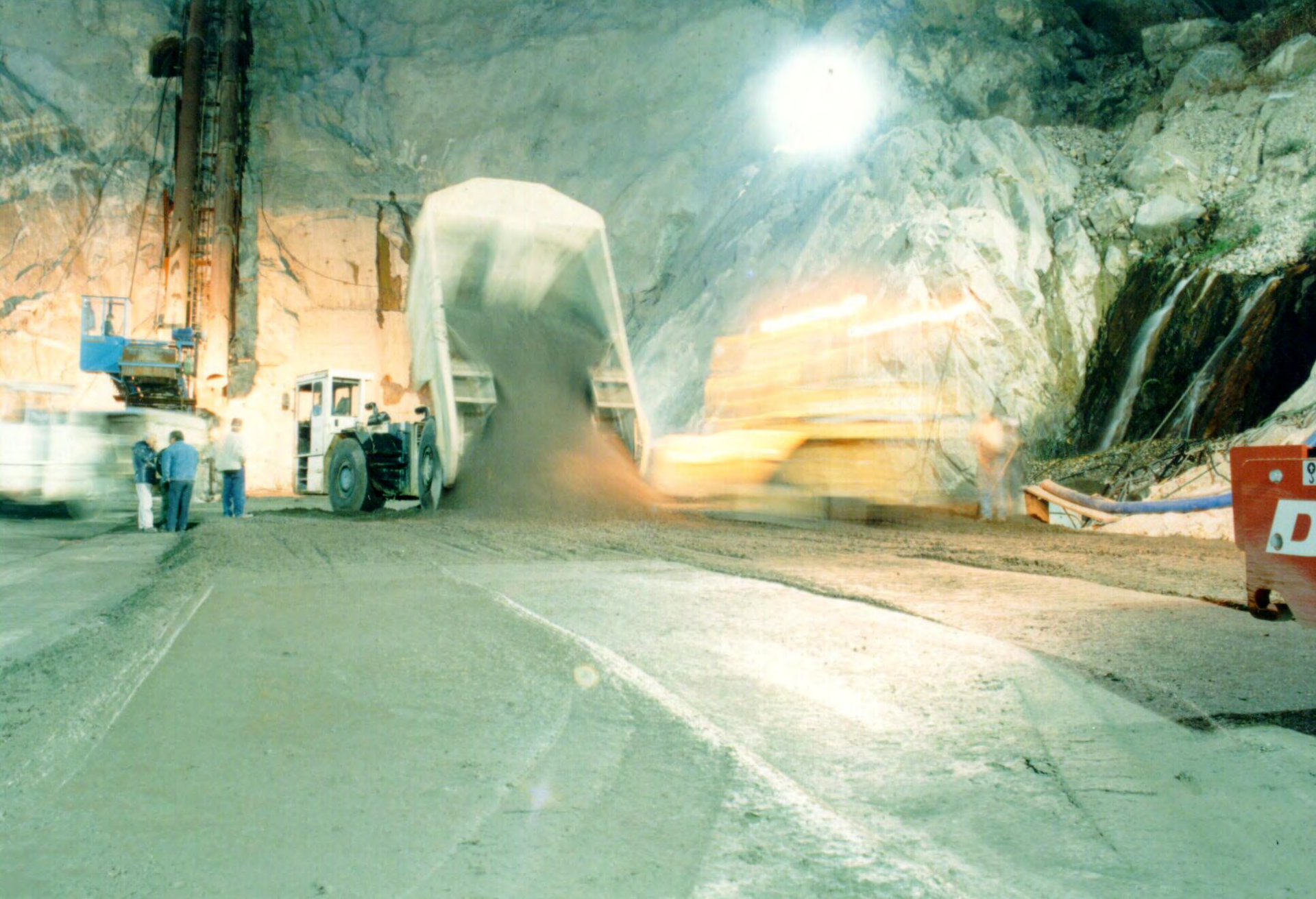
•RCC placement. Truck unloading.
