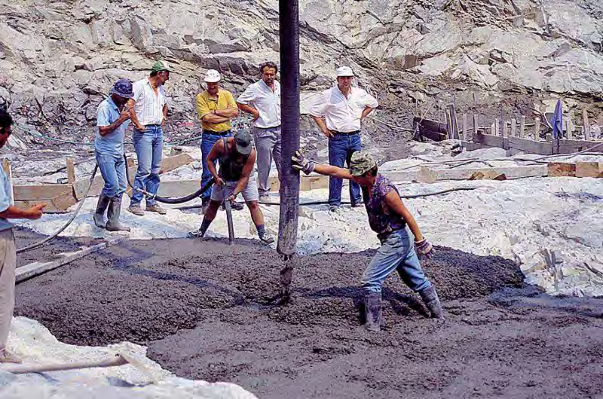
•Leveling concrete placement.
