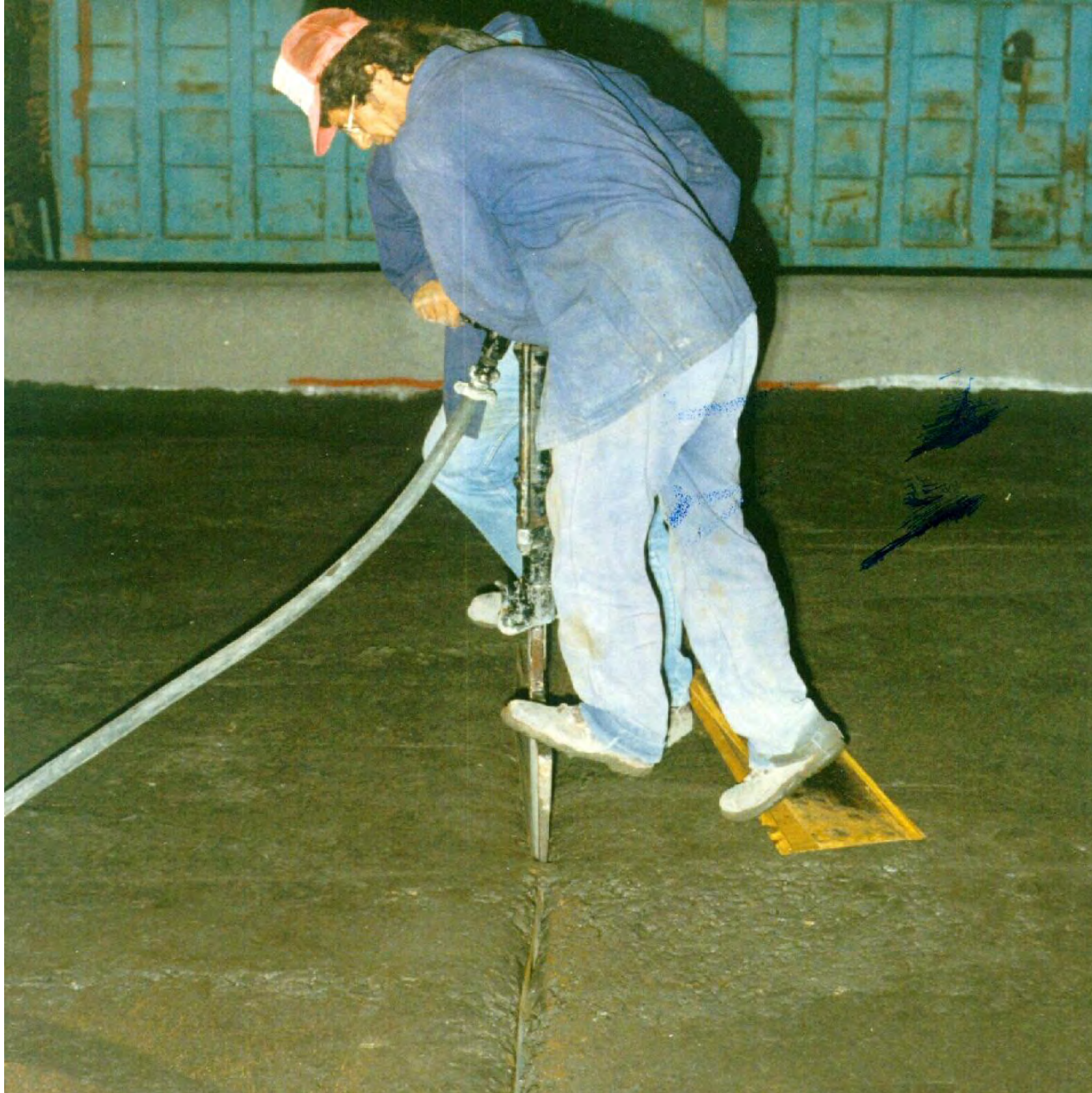
•Fabrication of joints. (Inserting separating steel blades).
