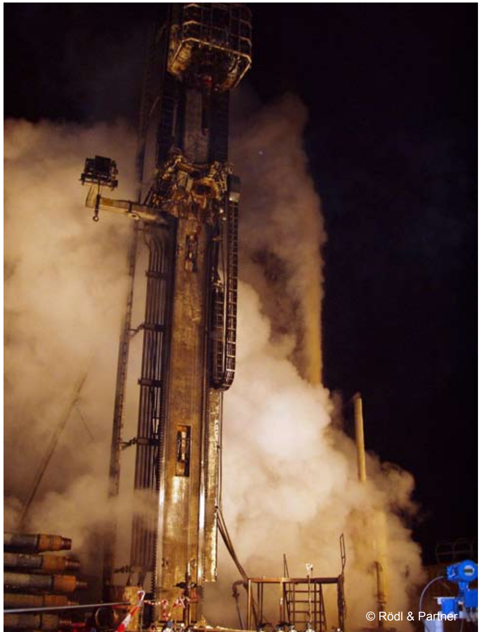
Pump test production drilling in Unterhaching, Germany
